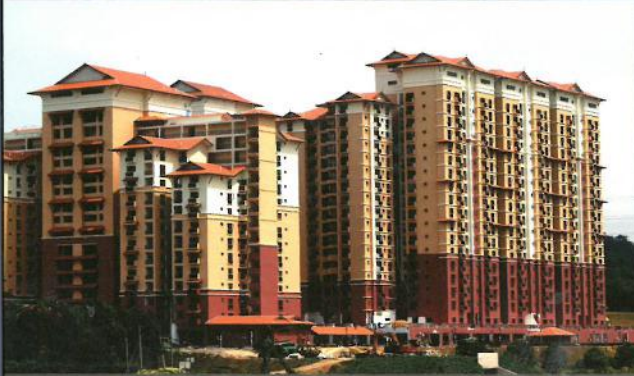
830 UNIT APARTMENT AT PUTRAJAYA
