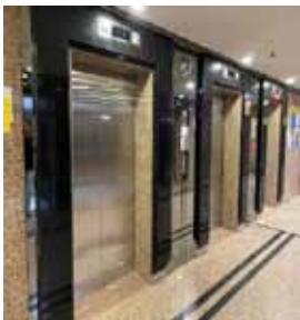
Lift Lobby & Lift Car
