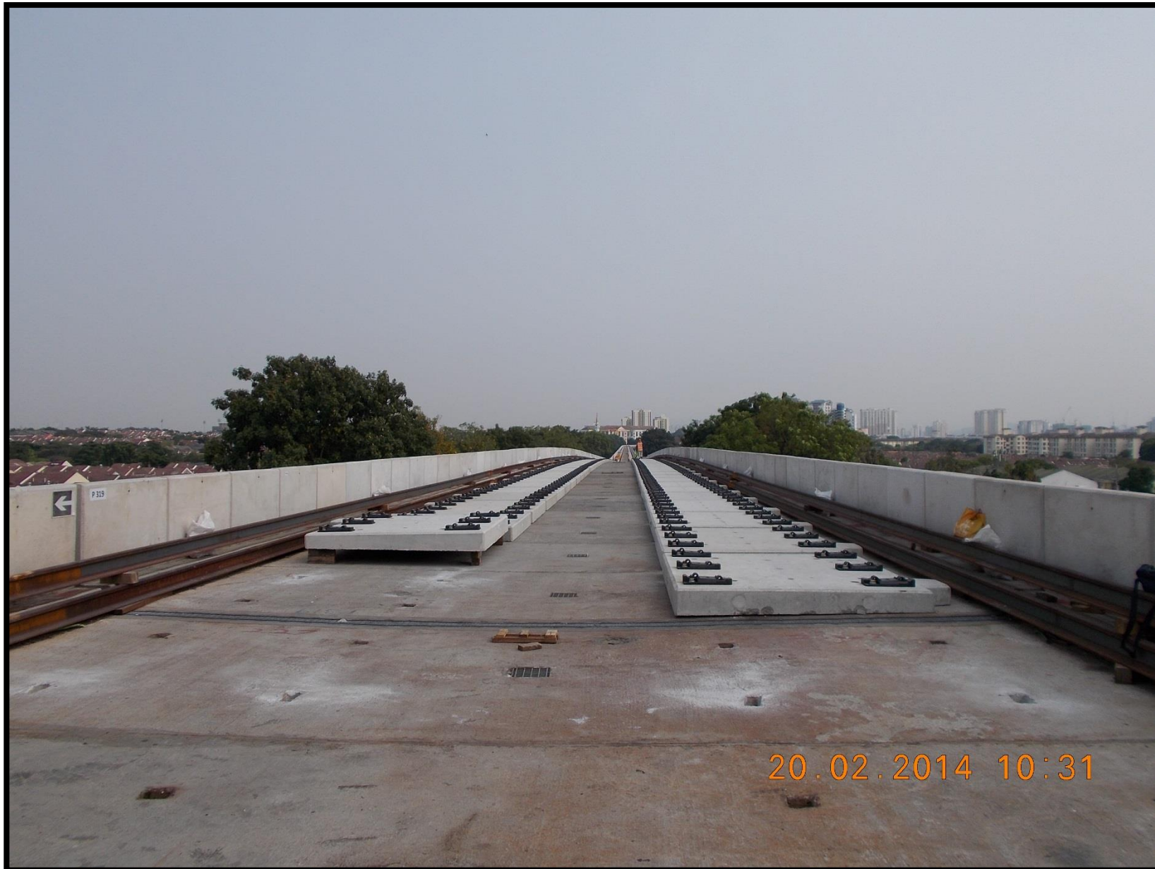
Positioning of precast sleepers.
