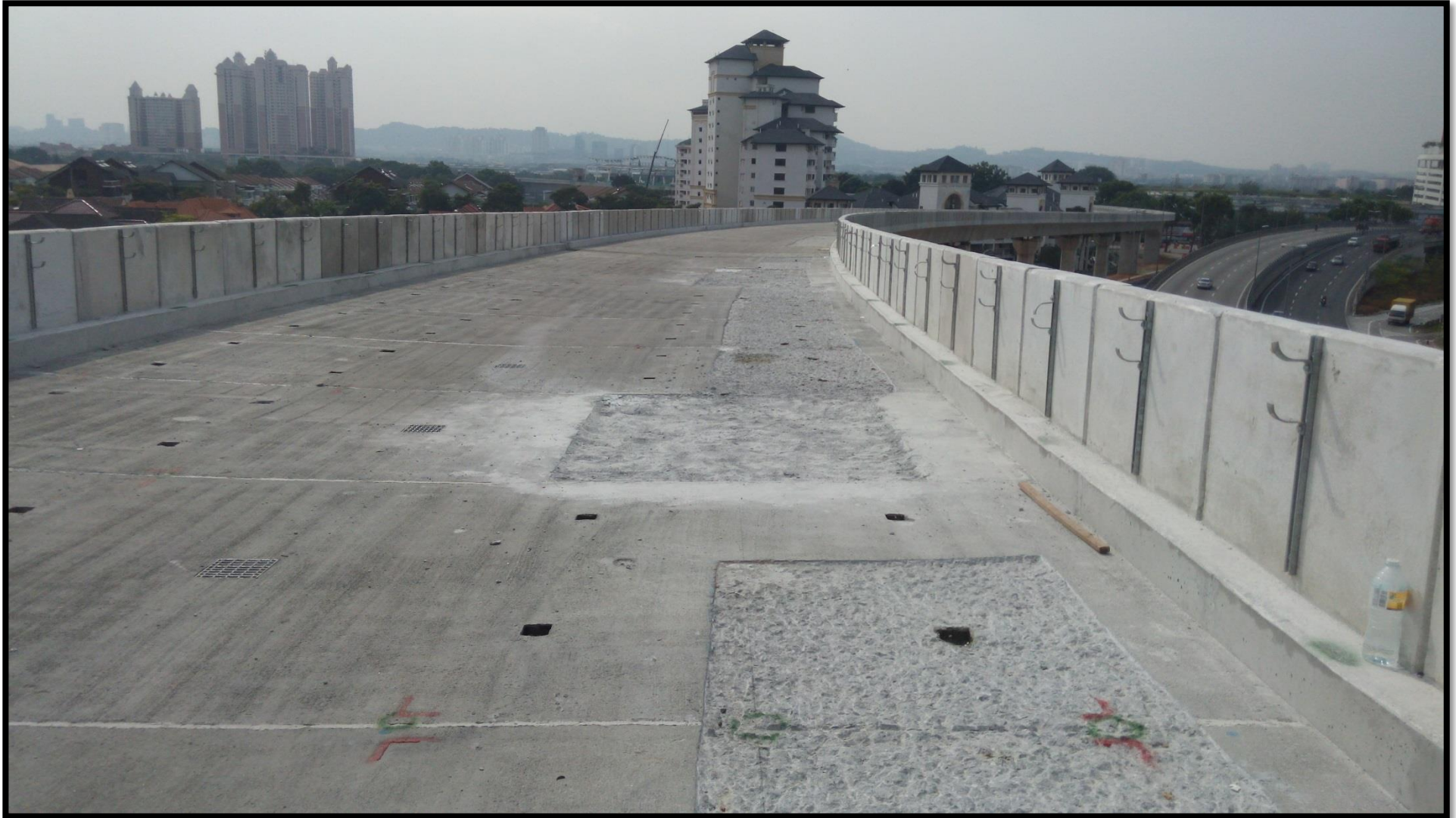
Guideway deck slab.
