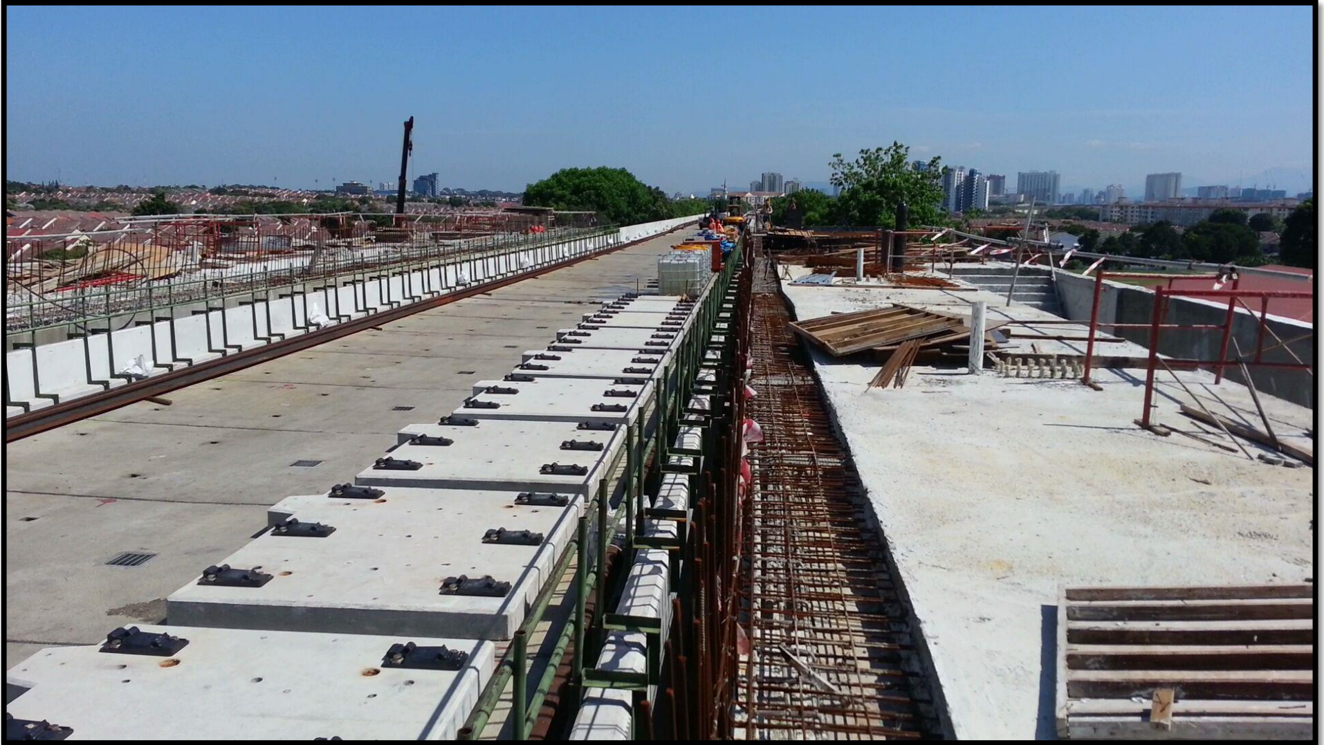
Casting of edge of platform after completion of track laying.
