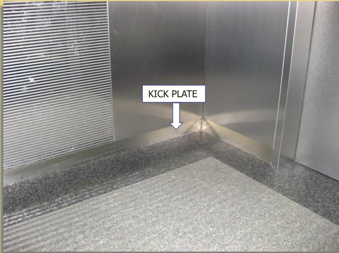
**Lift Car Shall Incorporate A Kick-plate At Least 100mm High At The Bottom Edges Of The Car Floor**
