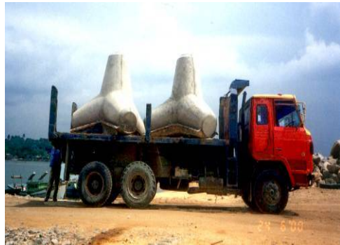
Transporting of breakwater
