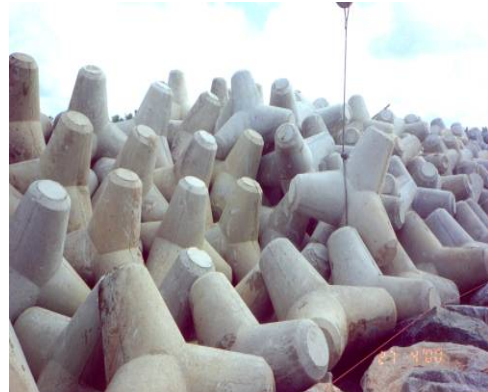
Placing of second layer of 3.8t tetrapod
