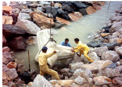
Placing of 3.8 t tetrapod
