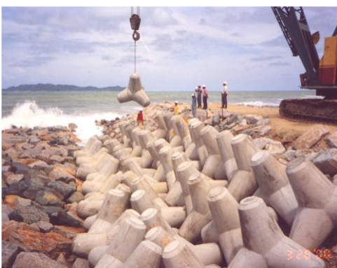
Placing of first layer of tetrapod
