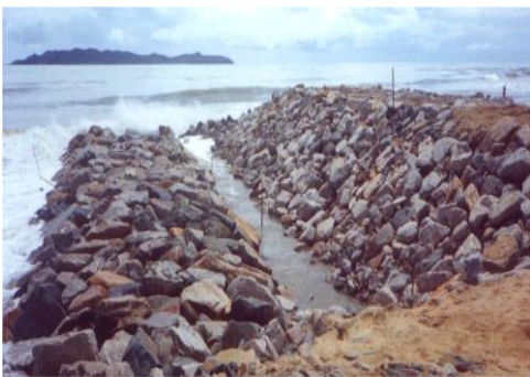
Toe Berm & Filter layer nearing completion
