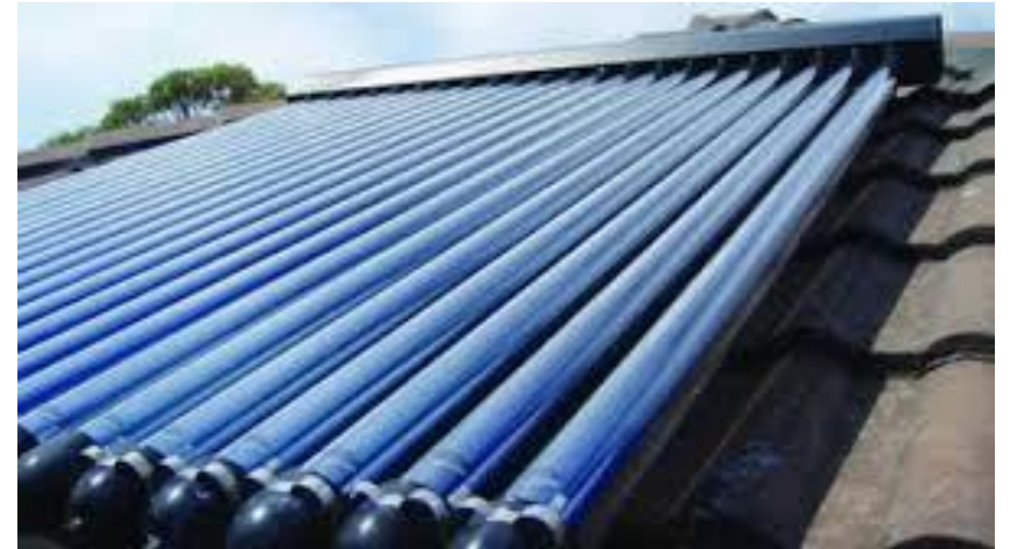
Solar evacuated tube
