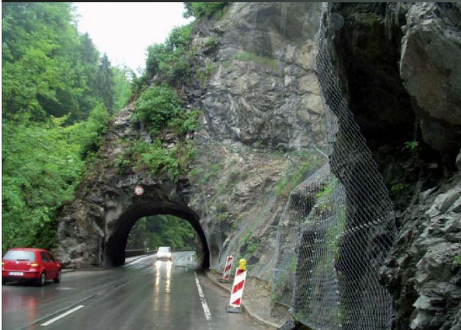
TECCO® drappe in June 2005 after installation; Ramsau Germany (after Geobrugg AG)
