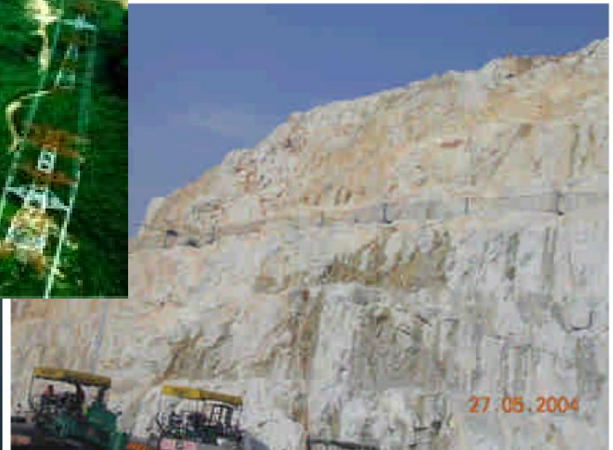
Photo 2 : Completed Geobrugg Rock Fall Fence at 20m Wide Berm
