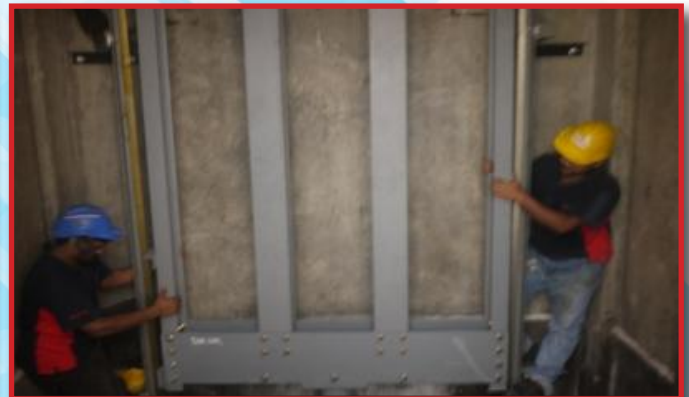
▲ Kerja memasang counterweight frame
