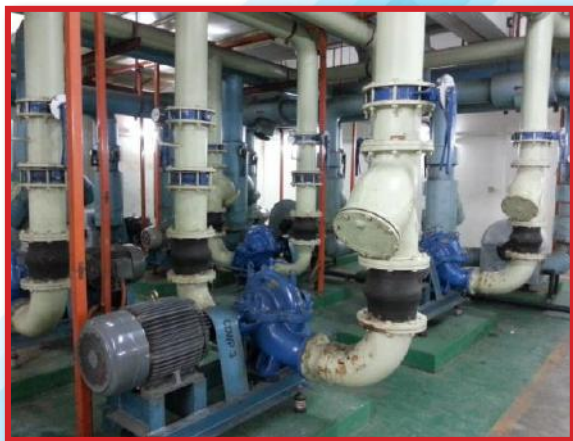
▲ Pump, piping dan fitting lama
