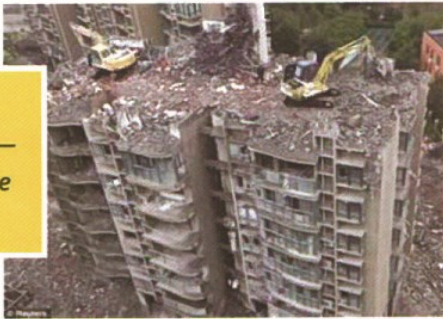
Mechanical Method by Hydraulic Crushers
