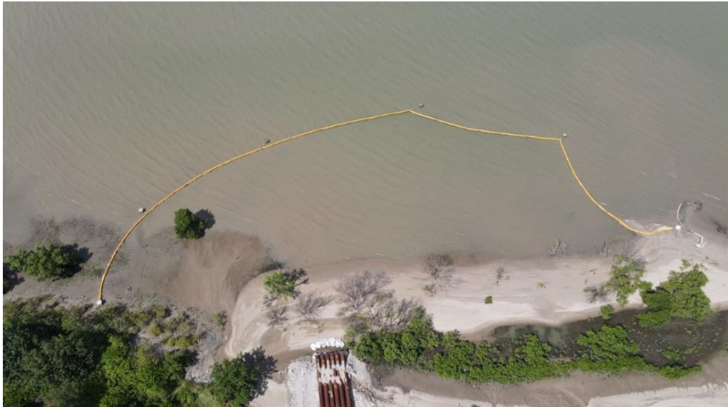
Silt Curtain enclosing Discharge Outlet System
