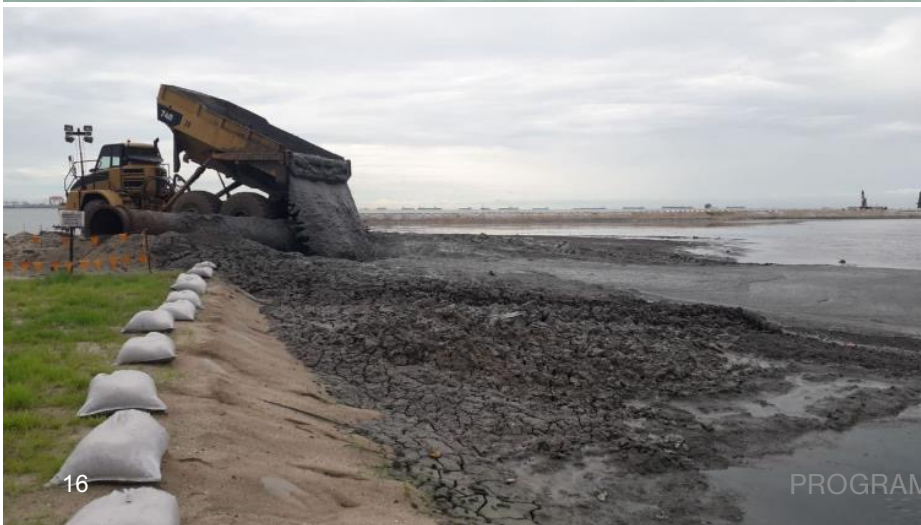
Dump truck tips dredge material into the bund
