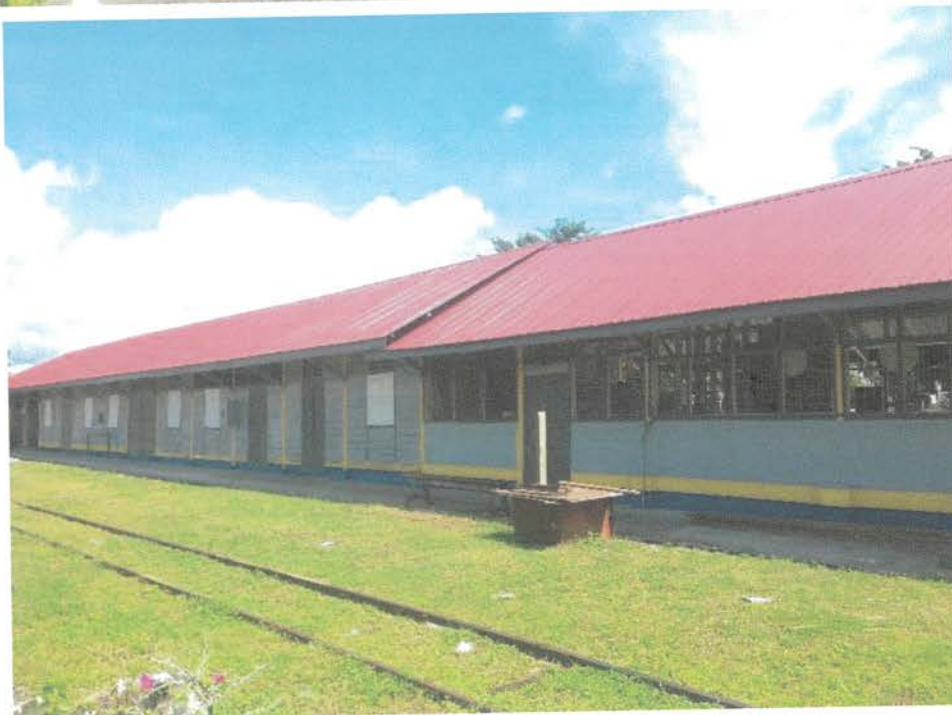
Foto 16: Bangunan KTMB Facility Management Office and Store
