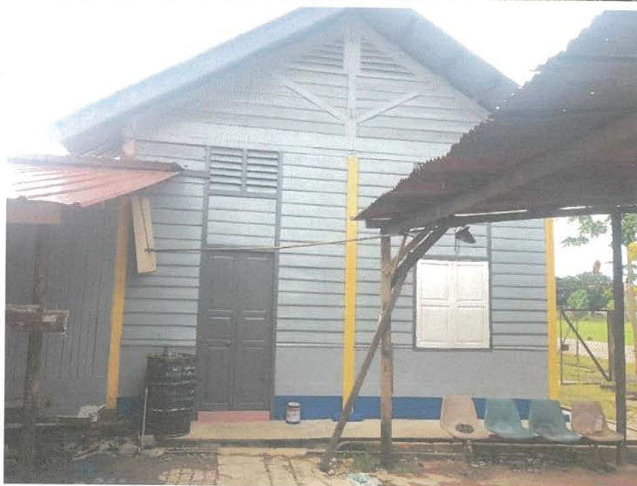
Foto 17: Bangunan KTMB Bridge Technician Office
