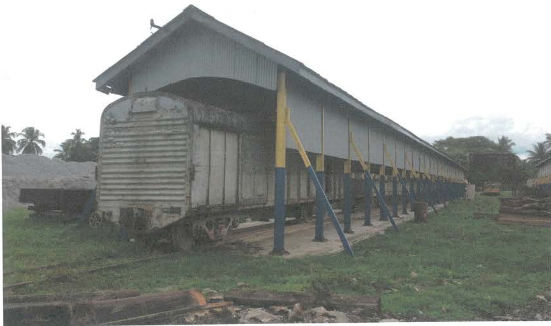
Foto 19: Bangunan KTMB Carriage Shed
