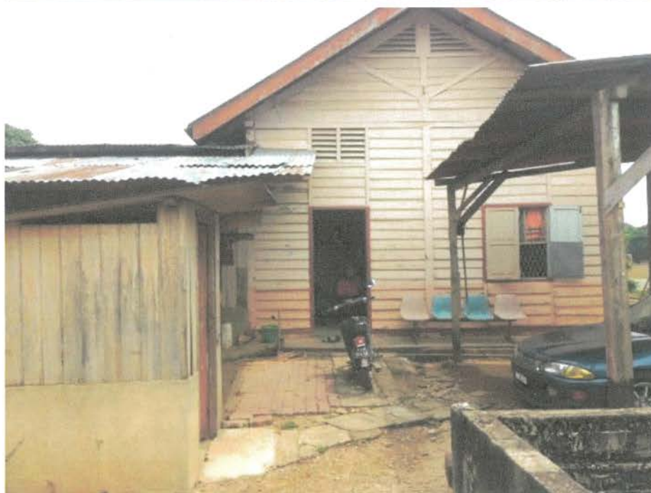
Foto 5: Bangunan KTMB Bridge Technician Office
