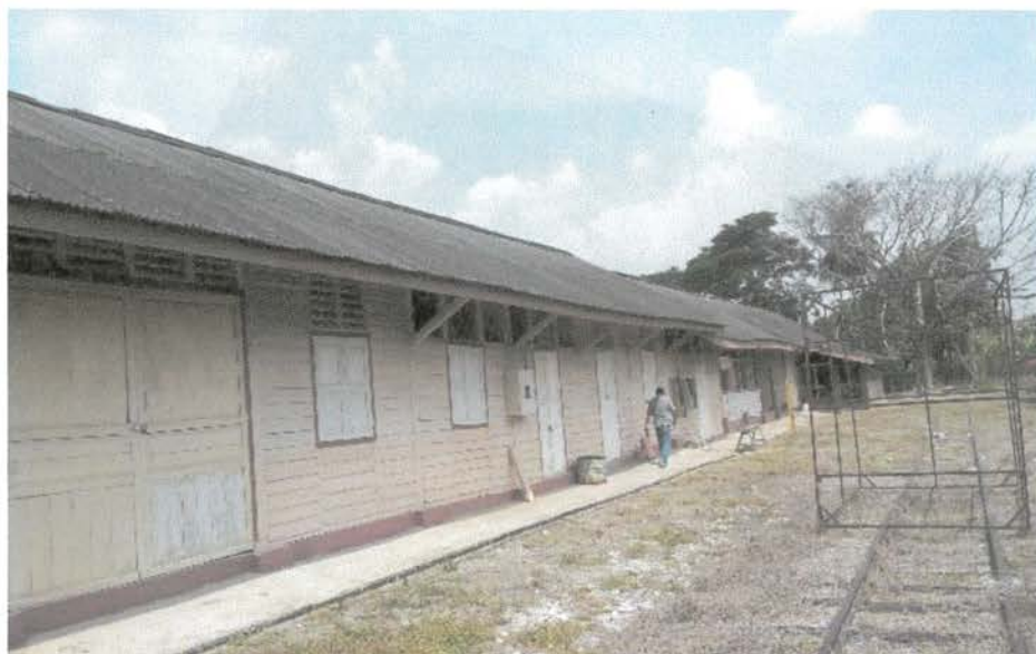
Foto 4: Bangunan KTMB Facility Management Office and Store
