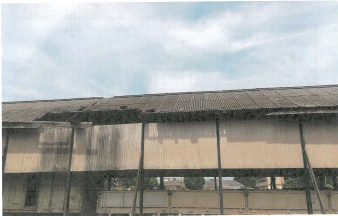
Foto 7: Bangunan KTMB Carriage Shed
