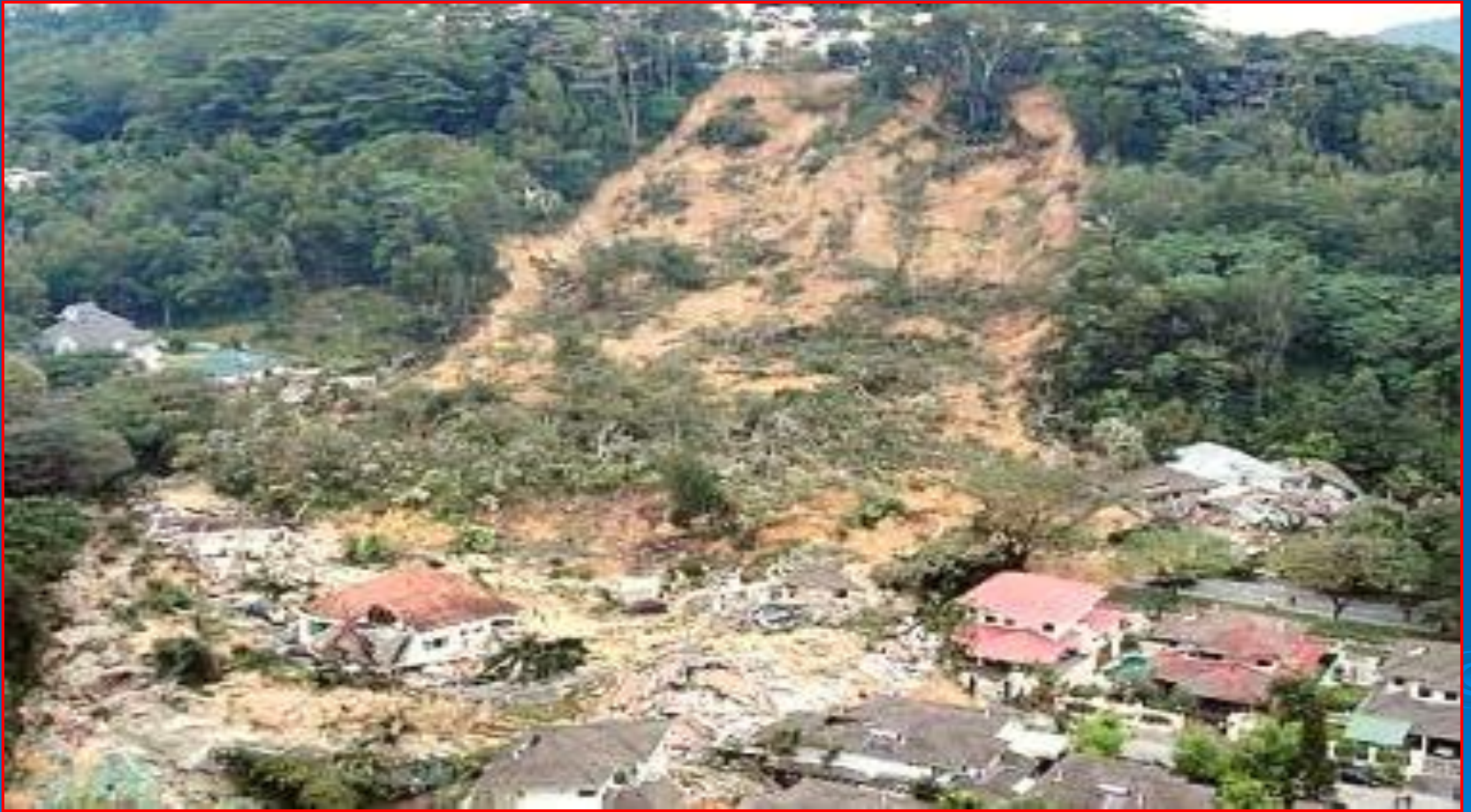
View of Bukit Antarabangsa Landslide
