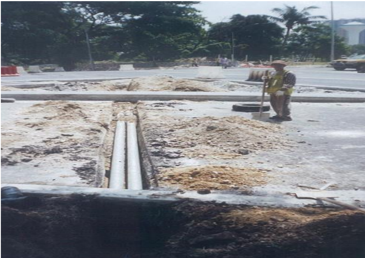
Laying G.I Pipe on Carriageway
