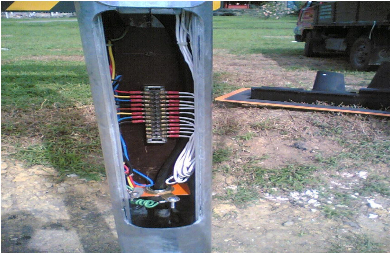
Termination Signal Cable On Traffic Pole
