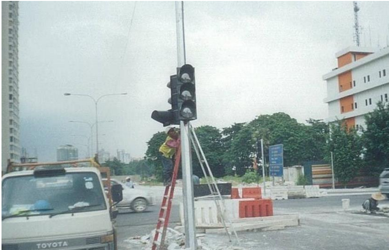
INSTALL TRAFFIC SIGNAL ASPECT AT STREET LIGHTING POLE
