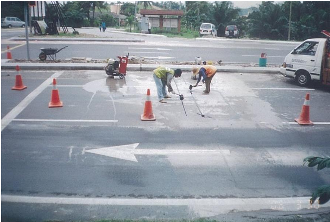
Install Traffic Signal Loop Detector
