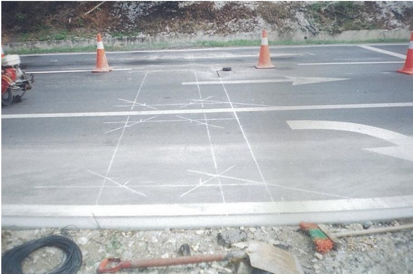
Install Traffic Signal Loop Detector
