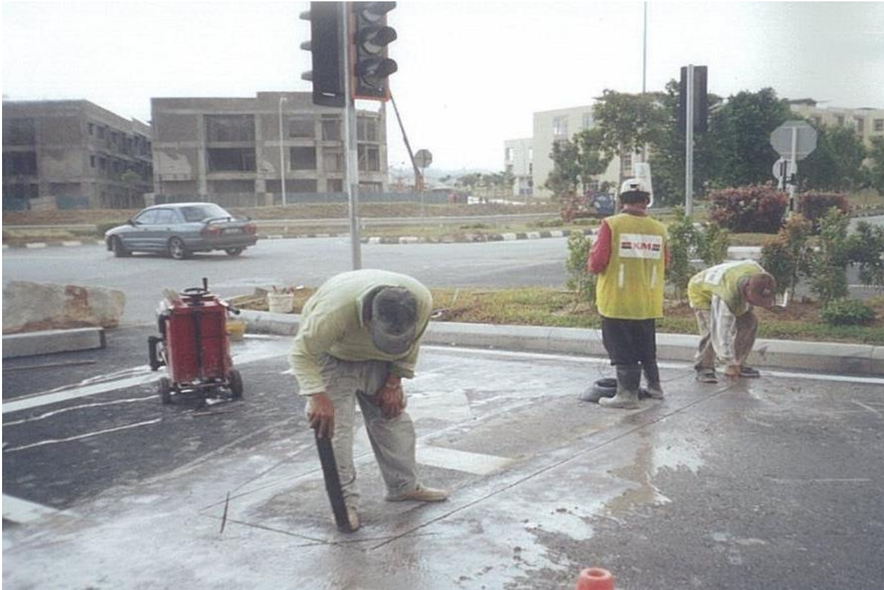
Install Traffic Signal Loop Detector
