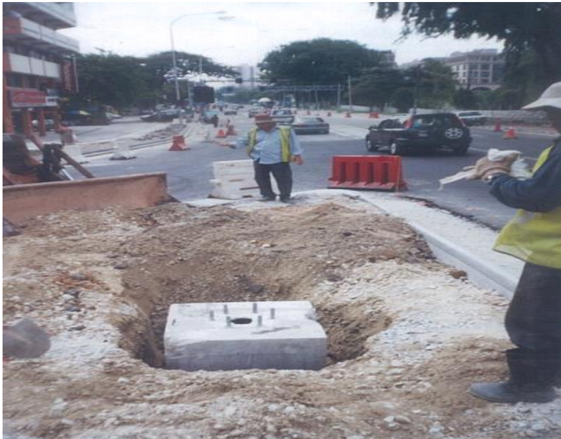
Traffic Signal Overhead Pole (Mast Arm) Plinth
