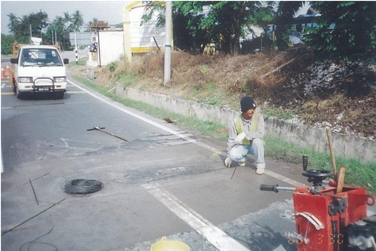
Install Traffic Signal Loop Detector
