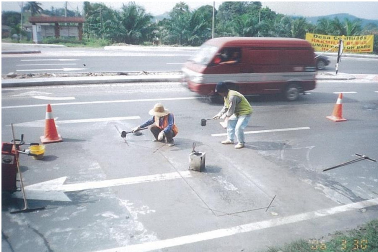
Install Traffic Signal Loop Detector
