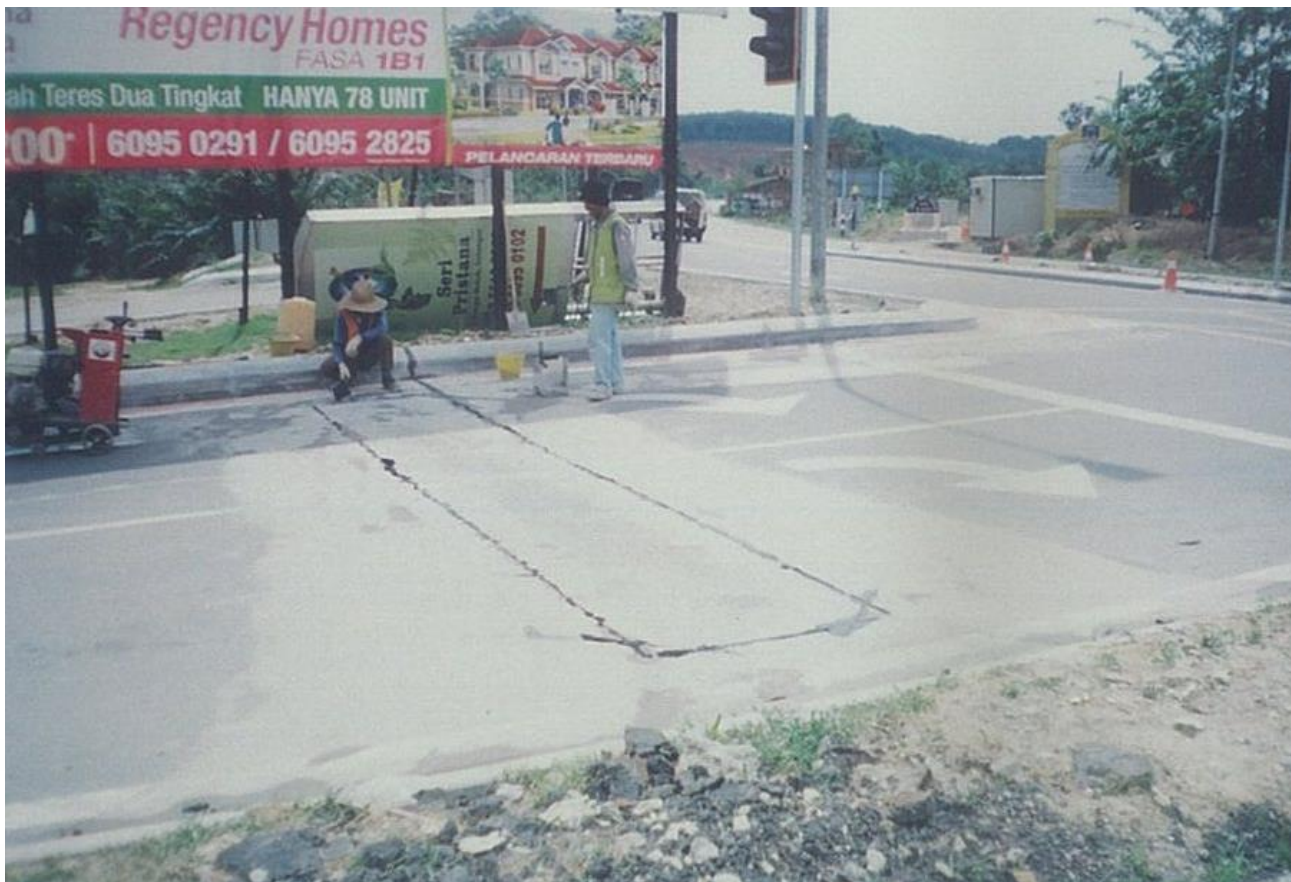
Install Traffic Signal Loop Detector
