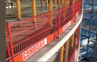
Sockets in slabs for edge panels
