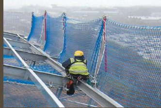
Holes in steel for net guards
