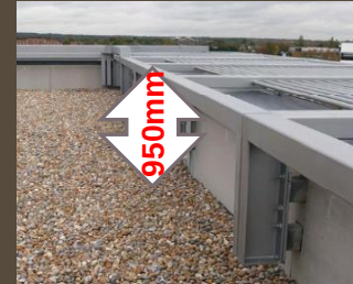
View of room upstand
