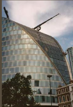
BMU Building Maintenance Unit
