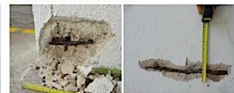
CONCRETE SPALLING
