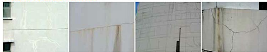
EFFLORESCENCE
