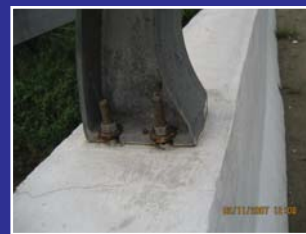
Anchoring bolts system for holding down cast iron posts at the railing system above the concrete parapet were not fixed properly.
