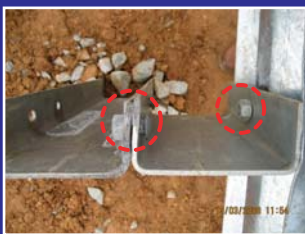
Quite a number of the g.i. bolts used to secure the corrugated guard rail were of insufficient protruding length.
