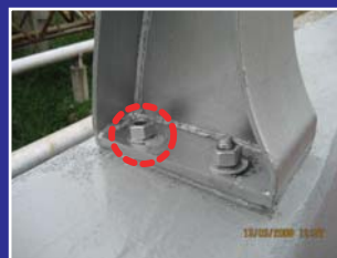
Anchoring bolts system for holding down cast iron posts at the railing system above the concrete parapet were fixed with anchor bolts of insufficient protruding length.
