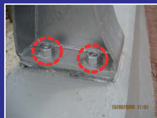
Anchoring bolts system for holding down cast iron posts at the railing system above the concrete parapet were fixed with anchor bolts of insufficient protruding length.
