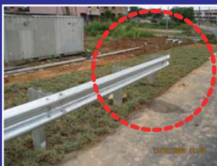
Wrong detailing of the end portion of the corrugated guard railing system.
