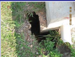
A big cavity was detected at the left side of the abutment B caused by effect of erosion.
