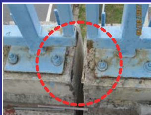
Joint sealants applied were either totally lost or partially detached.
