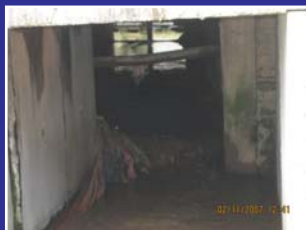
Wrong alignment of culvert extension causes the outlet choked with debris.
