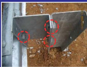
Quite a number of the g.i. bolts used to secure the corrugated guard rail were of insufficient protruding length.
