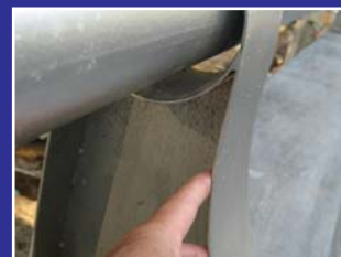
Sub-standard type of C.I. railing was used and fixed.
