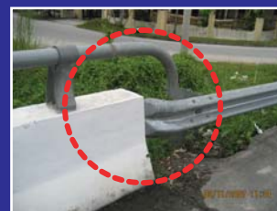
Detailing of corrugated guard railing system at the wingwalls portion were found to be fixed not according to the contract drawings.
