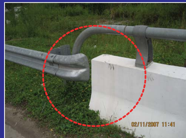
Detailing of corrugated guard railing system at the wingwalls portion not fixed according to the contract drawings. The spacing of the guard posts and end detailing not fixed to the requirements as in the contract drawings.
