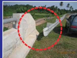
Detailing of corrugated guard railing system at the wingwalls portion were found to be fixed not according to the contract drawings.
