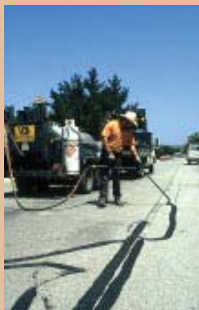
Crack sealing in the U.S.
