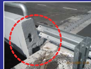
Detailing of corrugated guard railing system at the wingwalls portion were found to be fixed not according to the contract drawings.
