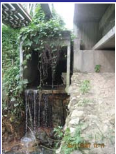
A big cavity was detected at the left side of the abutment B caused by effect of erosion.
