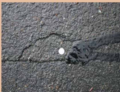
Crack sealing in Taiping, Perak.
