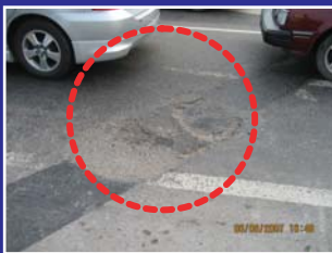
Expansion joint cracks, spalled and partly detached
