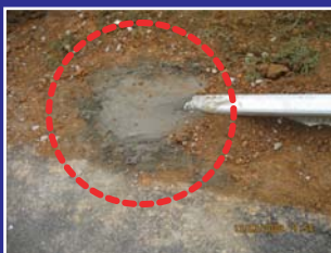
No proper concrete stump was provided as per construction drawing.
