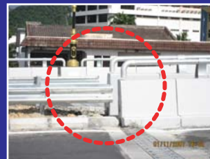
Detailing of corrugated guard railing system at the wingwalls portion were found to be fixed not according to the contract drawings.
