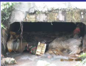
Existing service pipes were not removed, hence the stream flow was partially blocked.
