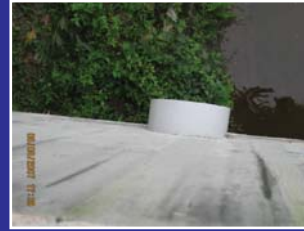
UPVC drain pipes having insufficient pipe length at outlet.
