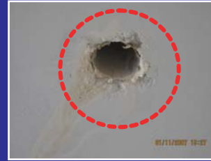
Inadequate extension drain pipe protruded length to soffit of box girder.
