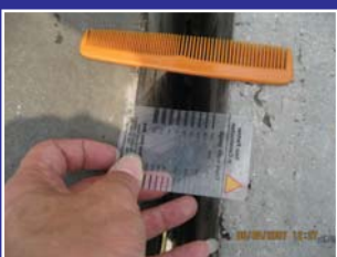
Expansion gap at mid span of the pedestrian bridge in front of S.M.K. Sg. Petani was found to be too big. ( \pm 55\text{mm} )
