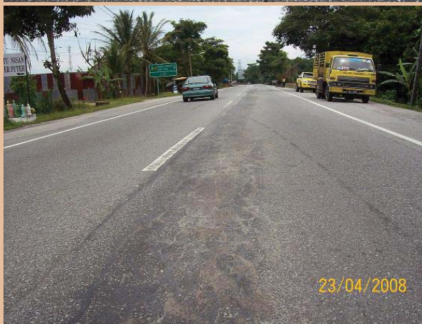
Crack sealing in Taiping, Perak.
