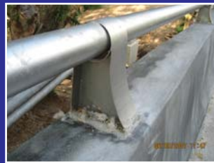
Sub-standard type of C.I. railing was used and fixed.
