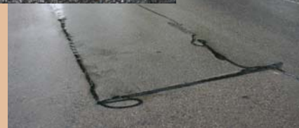
Crack sealing in Sydney, Australia.
