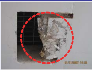
One of the manhole access to soffit of box girder was plug with residual mass concrete.
