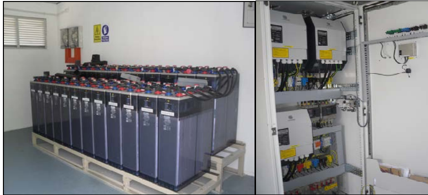
Figure 3.9 : 3500 Ah battery bank at SK Penontomon (left) and inverter (right) at SK Penontomon. (Source : Abdul Muhaimin Mahmud)
