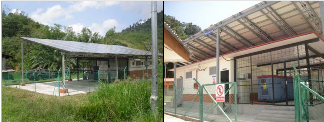
Figure 3.7 : Solar PV panel. (Left) 20 kWp at SK Penontomon, (right) 25 kWp PV and 40 kW diesel generator at SK Pulau Sepanggar. (Source : Abdul Muhaimin Mahmud)
