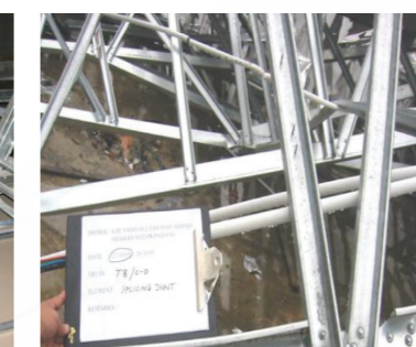
Web members at splicing joint
