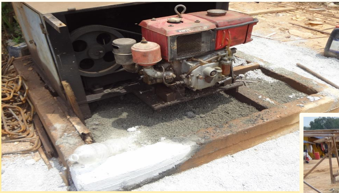
Containment Bund for bar bender
