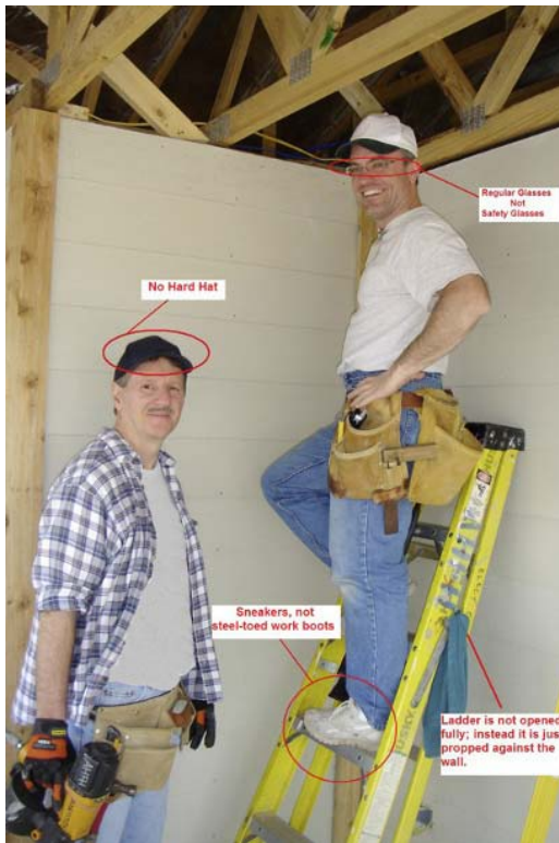
Figure 12.6 A spot inspection of this contractor's job site identified a number of safety infractions. The supervisor snapped this photo and then marked-up and posted the picture on the job site as a reminder for all employees to think about safety and practice safe work methods.
