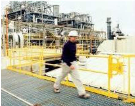
Utility Grid Switching
