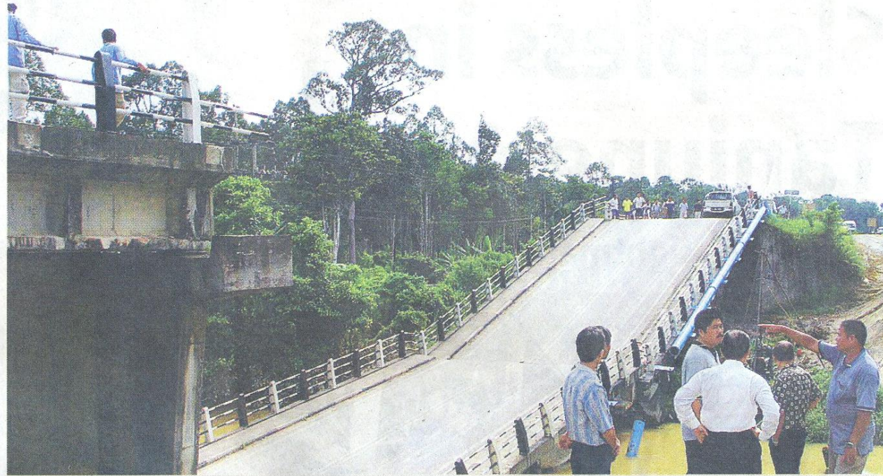
WRECKED: Residents inspecting the site of the broken bridge across Sungai Menyan in Kanowit yesterday.
