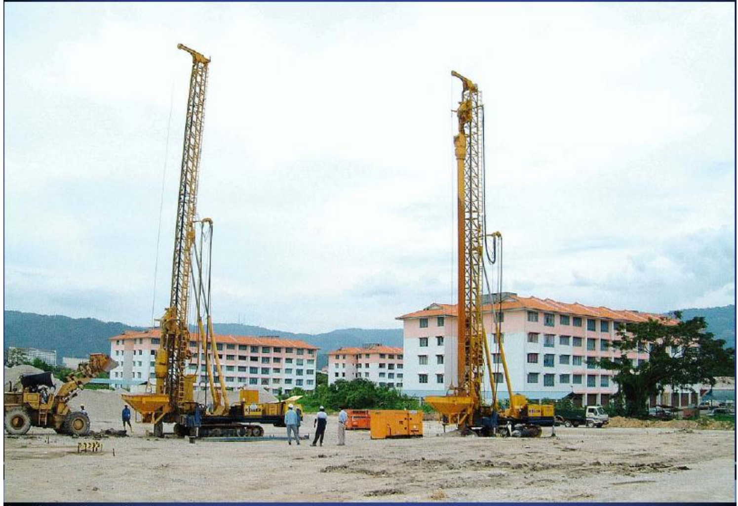
Vibro replacement at Jelutong Expressway
