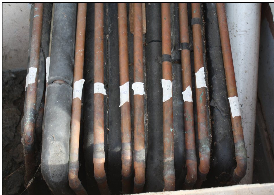
Gambar 9: Proses mengenal pasti pipe refrigerant .
