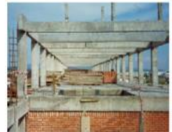
Monolithic rigid connection in reinforced concrete frames
