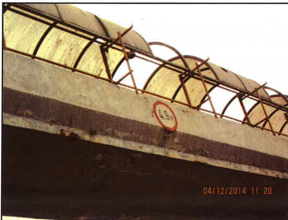
Gambar 25: Had Ketinggian Jejantas Sub-standard - papan tanda had ketinggian 4.9 m
