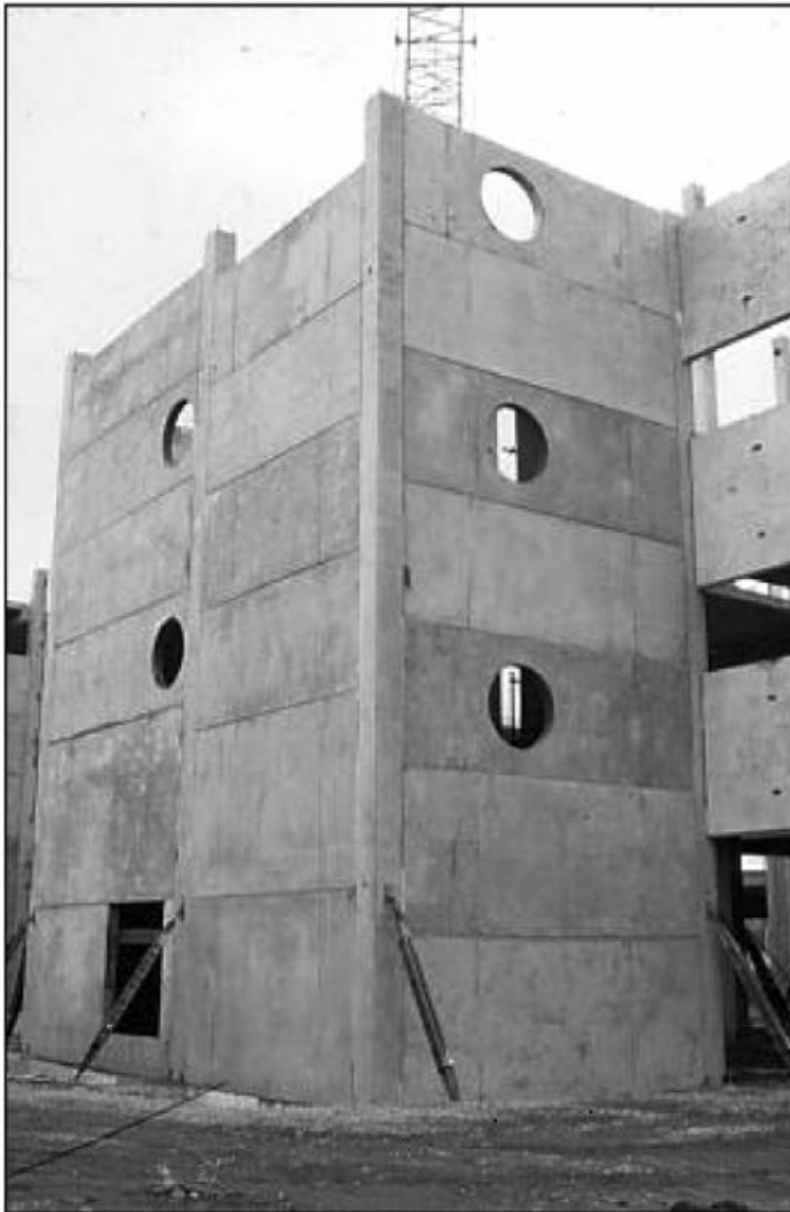
Precast concrete infill shear walls
