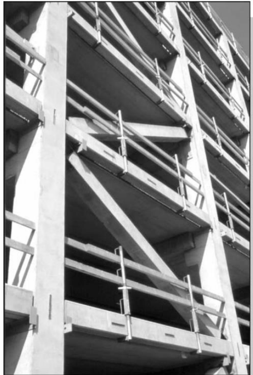
Precast concrete cross bracing
