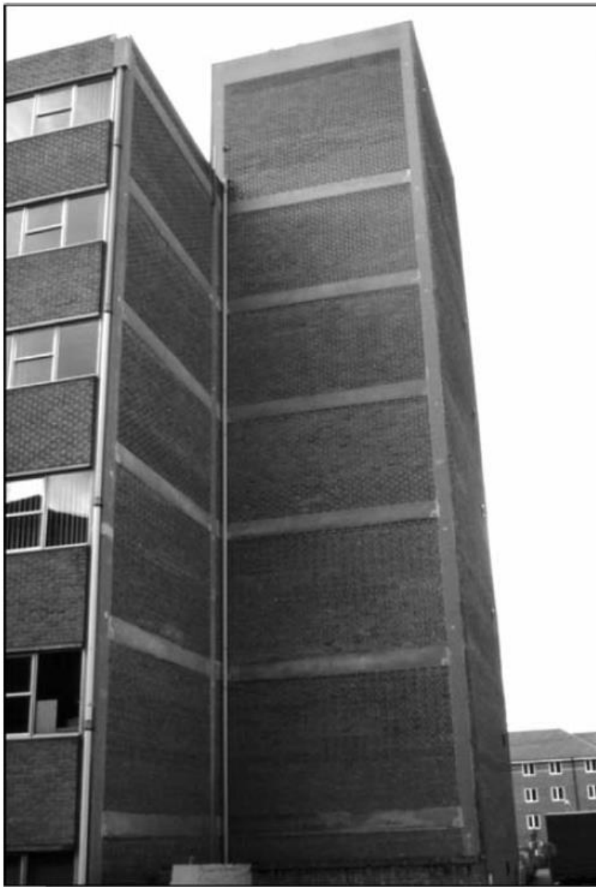
Brick infill shear wall.
