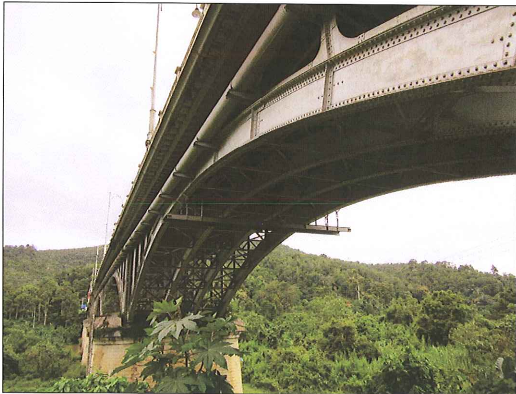
Picture 3 & 4 : General North-East views of Jambatan Sultan Iskandar Kuala Kangsar.
