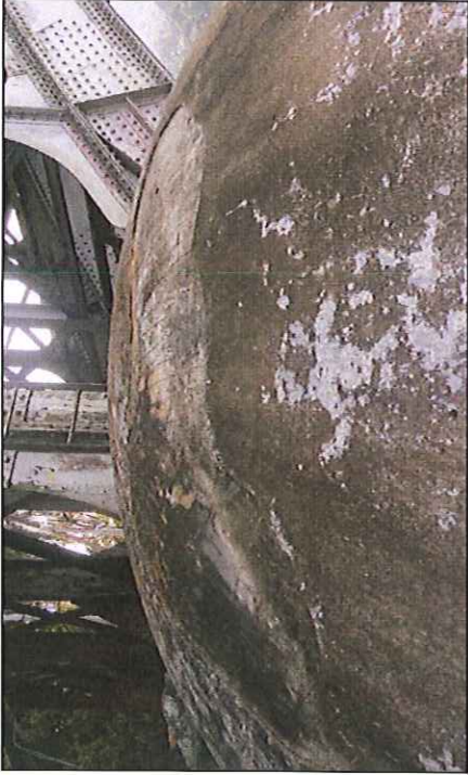
Picture 17 – Pier 6 (toward Kuala Kangsar)
