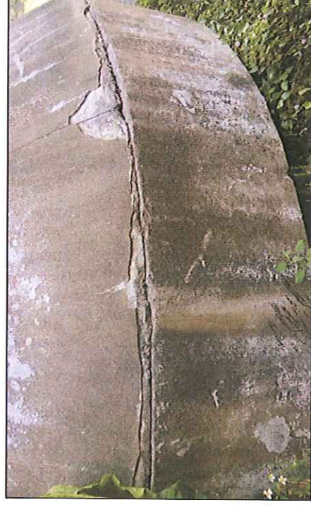
Picture 16 – Pier 6 (toward Kuala Kangsar)
