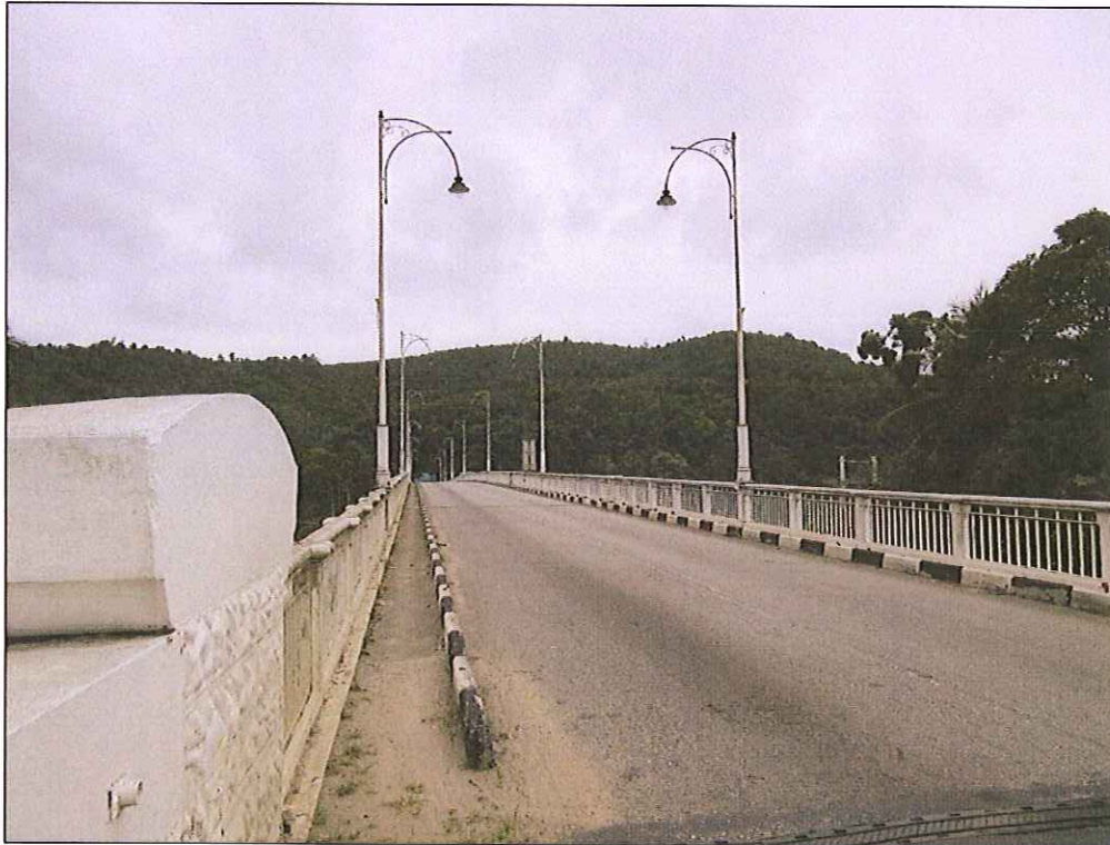
Picture 5 : General view of the North-West end of the bridge.
