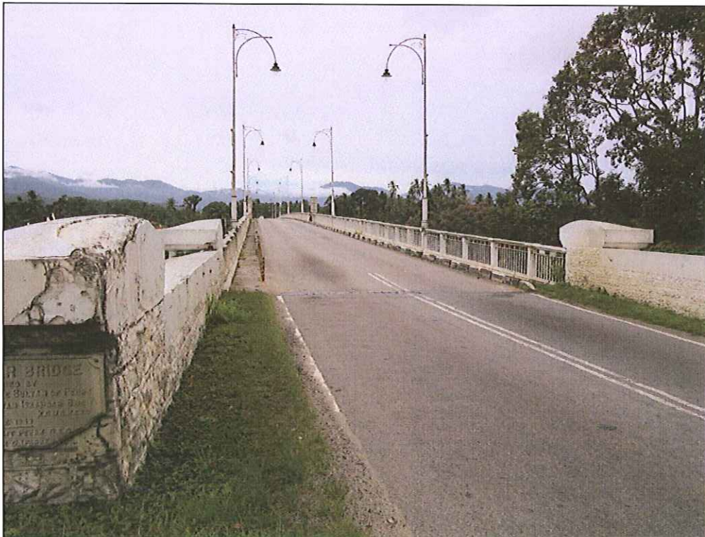
Picture 6 : General view of the South-East end of the bridge.
