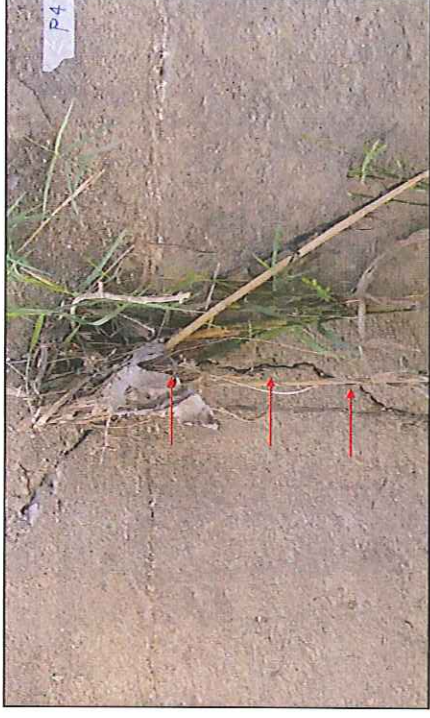
Picture 11 – Pier 4 (toward Kuala Kangsar)
