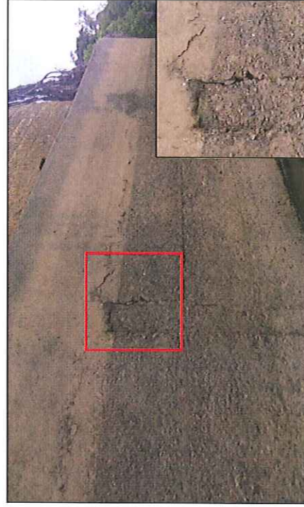
Picture 4 – Pier 1 (toward Kuala Kangsar)
