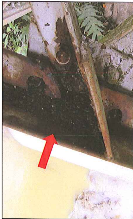
Picture M – S5 – P17 Moderate corrosion and rivet head deteriorate on inclined cross bracing.
