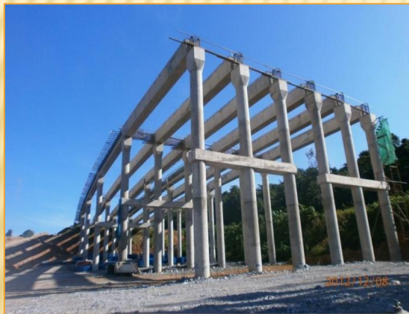
Disember 2012 - Construction Eco Bridge in Progress
