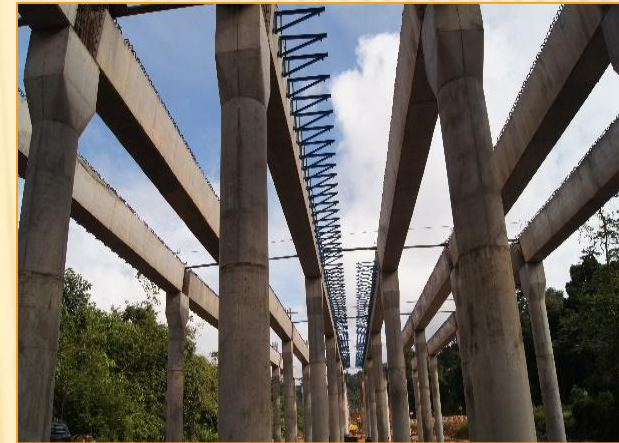
11 Jan 2013 – Rib Beams Installed
