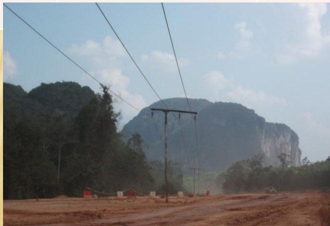
3E2 – Merapoh Relocation 33KV
