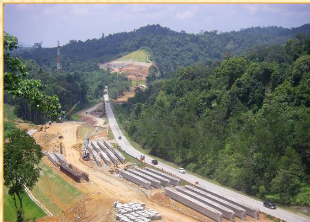
5 Apr 2012 – Beams and Parapets are being pre-cast adjacent to bridge site
