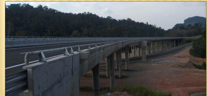
Eco Bridge No. 2 Seksyen 3F1.
