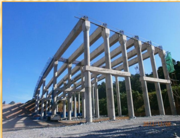
Disember 2012 - Construction Eco Bridge in Progress
