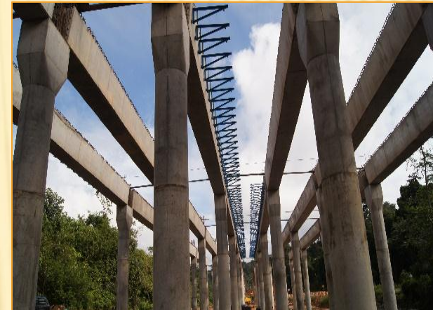
11 Jan 2013 – Rib Beams Installed
