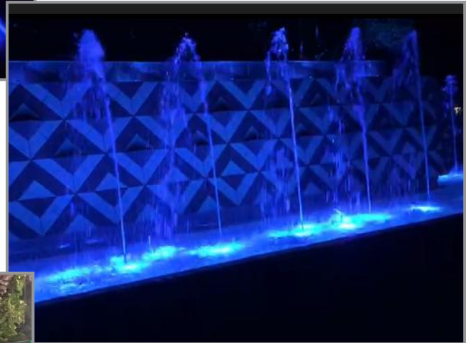
Trumpet jet with LED under water light ▶
