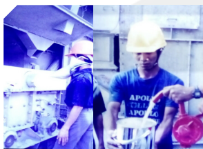
1993 @ Jalan Rembau Tampin - Adding Rubber Powder into the mixes
