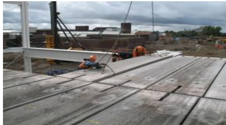
Precast floor slabs
