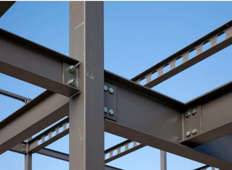
Steel beams and columns
