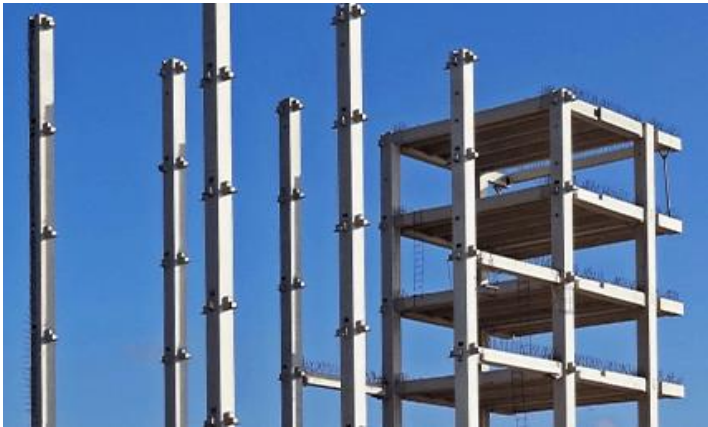
Precast beams and columns
