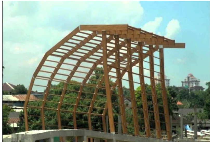
Fabricate timber frame ( glulam)
