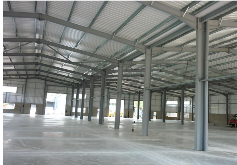
Steel portal frames
