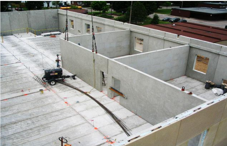
Precast concrete walls
