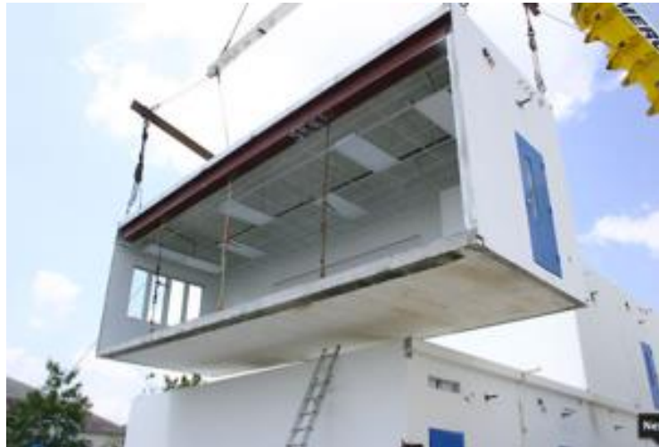
Precast concrete boxes
