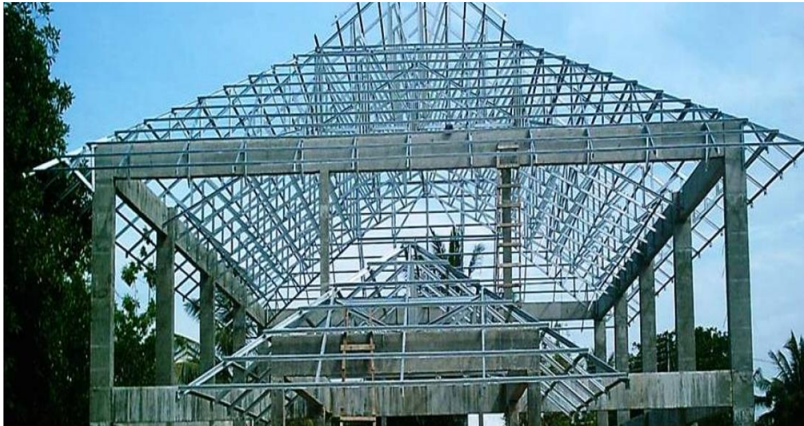
Steel roof truss ( Hot roll/ cold formed)
