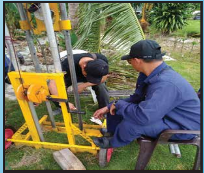
Rajah 7: Kerja-kerja Motorized JKR Probe dijalankan
