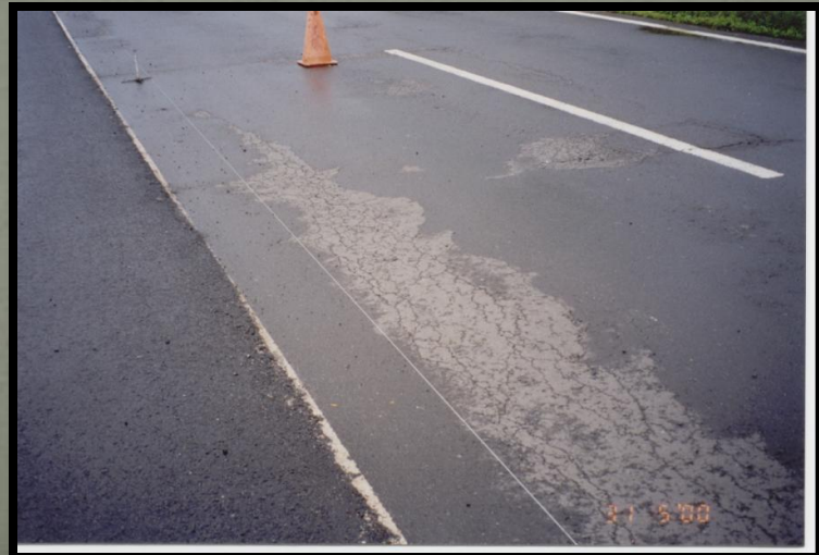
Shallow pavement distress
