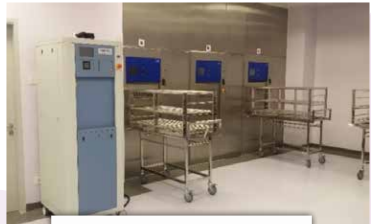
Sistem Pensteril Di Central Sterile Services Department (CSSD)
