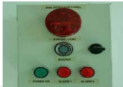
Gas Leak Detector Dan Gas Detector Panel Di Makmal
