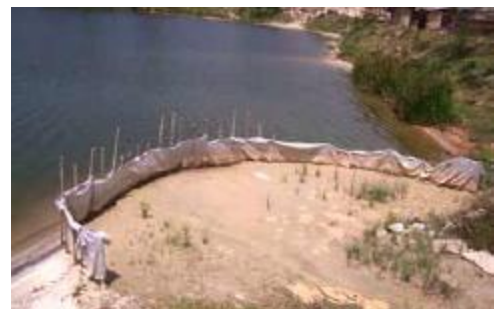
Figure 3: Silt Fence in Sediment Basin for Ease of Maintenance
