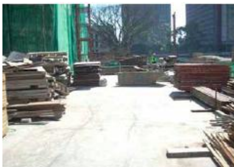
Figure 6: Materials Organized On Site According to Usage Frequency
