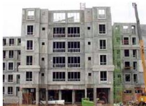
Figure 12: Precast walls – waste minimization via industrialized building system (IBS)
