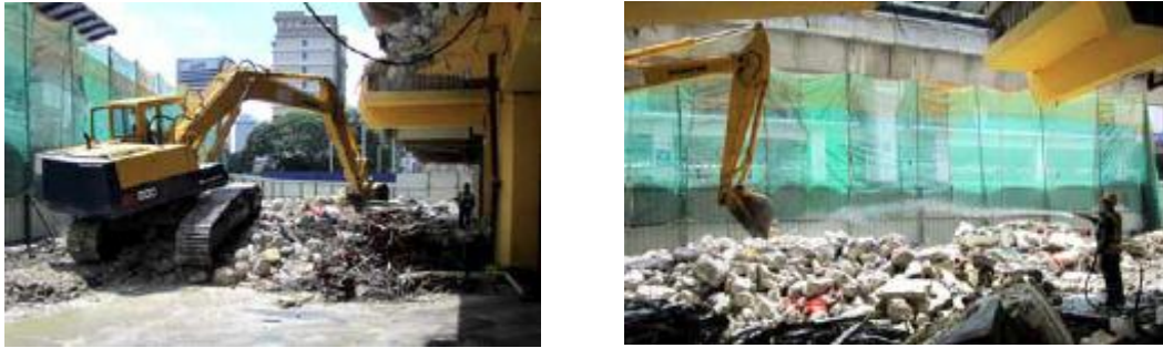
Figure 13: Concrete and Steel Bars from Demolition Works Are To Be Segregated For Recycling
