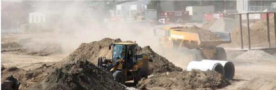
Figure 9: Poor Air Quality Due To Absence of Dust Control Measures
