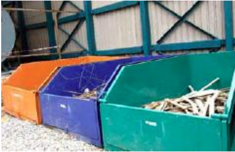
Figure 10: Provide Segregation Bin Construction Waste
