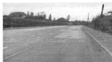
Fig. 2 — Rubberized bitumen surface-dressing experiment: cutback bitumen (background) at 4½ sq. yd/gal has fatted up; rubberized bitumen (foreground) at 4½ sq. yd/gal is in fairly good condition. (R.R.L., U.K. photo crown copyright reserved; reproduced by permission of the Controller, H.M.S.O.)
