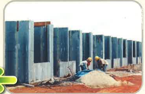
ERECTED ACOTEC PANEL WITH DOOR & WINDOW OPENING
