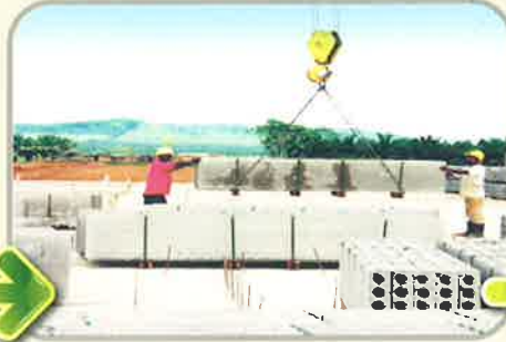
UNLOADING OF ACOTEC PANEL
