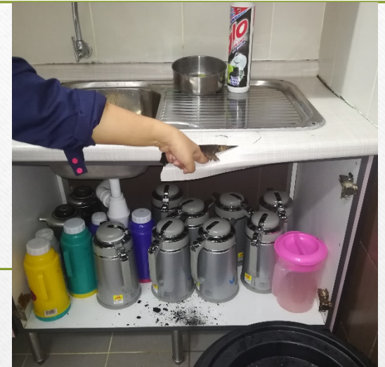
Sink top with HPL finished (not accordance with spec)
