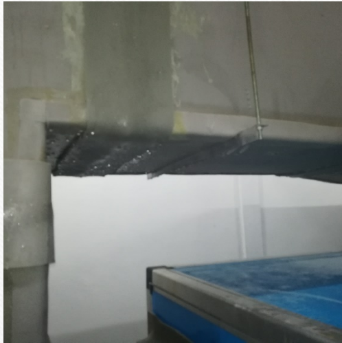
Condensation at air Cond duct without / improper insulation
