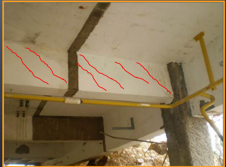
Shear failure
