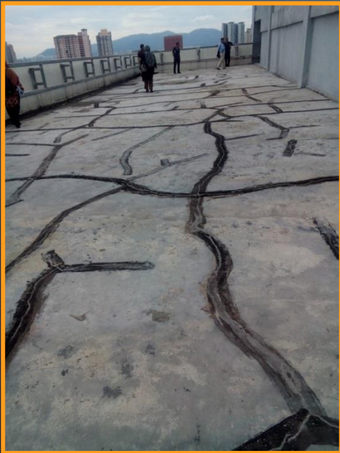
Plastic shrinkage cracks
