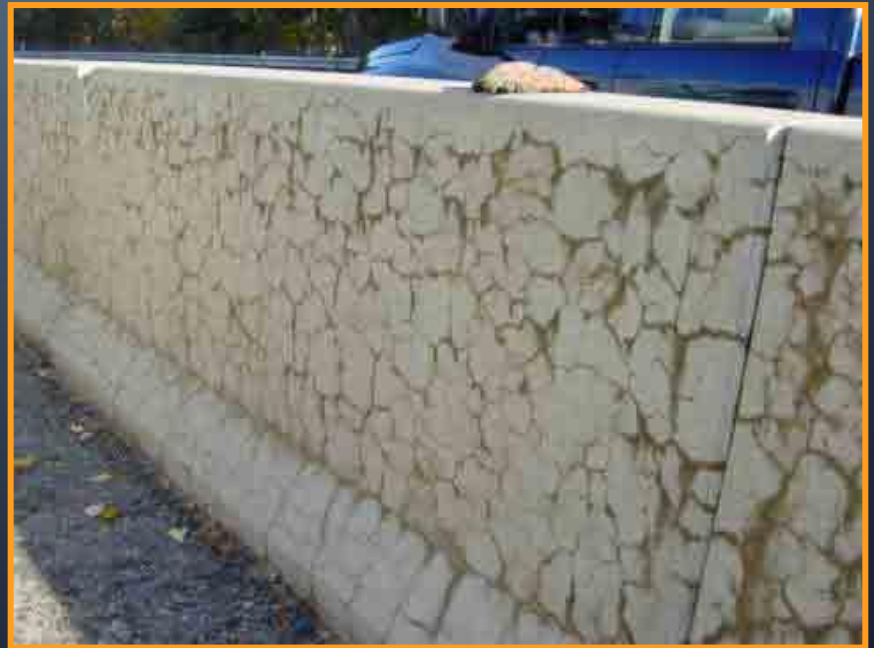
Alkali-aggregate reaction
