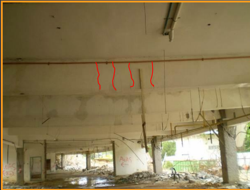
Bending failure
