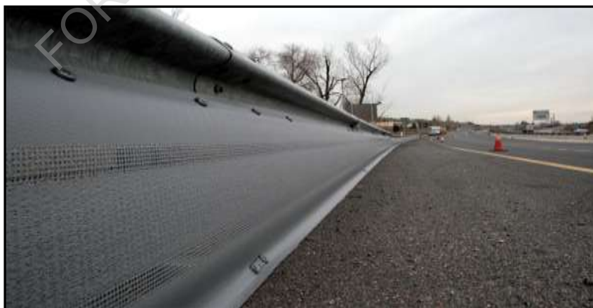
Figure 8.5: Photograph of Basic Motorcyclist Protection System (MPS) Fitted to the Existing Barrier System (Source: Cegasa Internacional)
