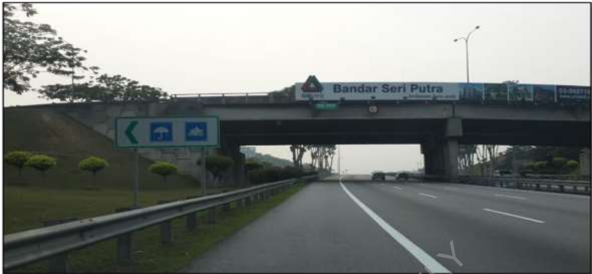
Figure 6.2: Under Bridge Motorcycle Shelter
