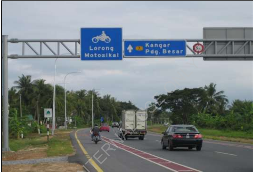
Figure 4.2: Example of Non-Exclusive Motorcycle Lane to be added onto Existing Roadways
