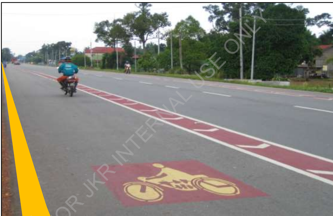
Figure 4.1: Example of Non-Exclusive Motorcycle Lane (Location: Federal Route 5, Jalan Abdul Rahman - Parit Jawa, Muar, Johor, JKR Malaysia)
