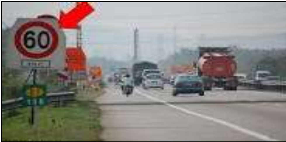
Inadequate number of advance warning signs
