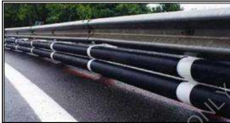
Figure 8.4: Photograph Of "Mototub "Fitted To Existing Barrier System (Source: Sodirel)
