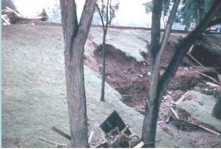
Erosion at the Downstream Face of Dam
