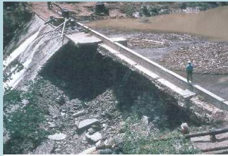
Erosion due to Dam Overtopped
