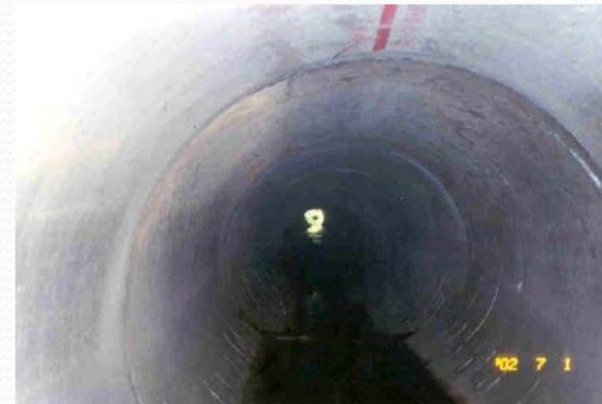
Surface undulations on the inside of culvert
