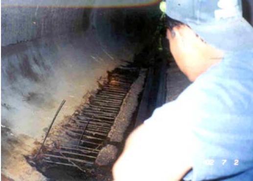
Failure at the bottom of culvert
