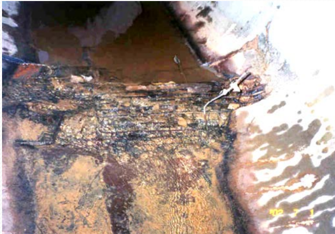
Failure at the bottom of culvert
