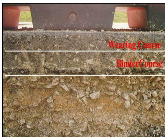
Rajah 4.7.3.1 : Wearing dan Binder Laying
