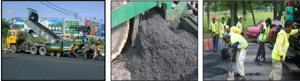
Rajah 4.7.3.3 : Proses Laying
