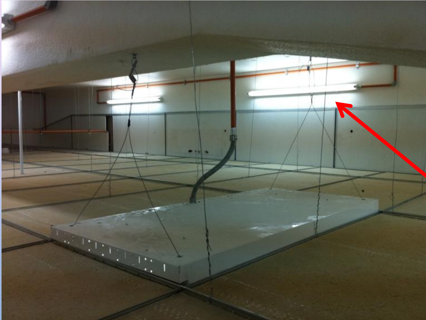
1 x 28W (T5) wall mounted bare channel
