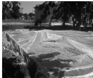
Using plastic sheet to cover concrete
