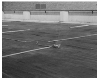
Wetting by water sprinkler
