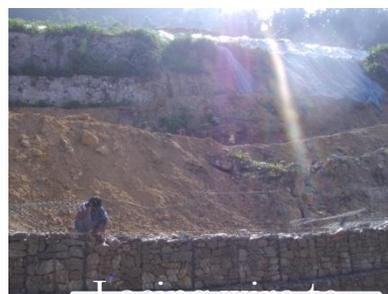
Lacing wire to tight gabion cage
