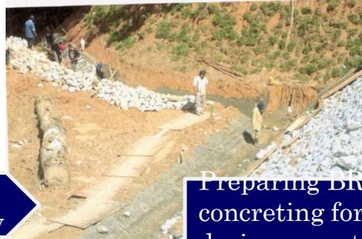
Preparing BRC & concreting for surface drainage system
