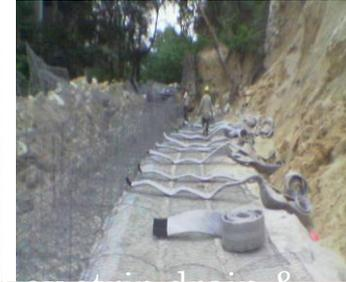
Lay strip drain & gabion cage preparation
