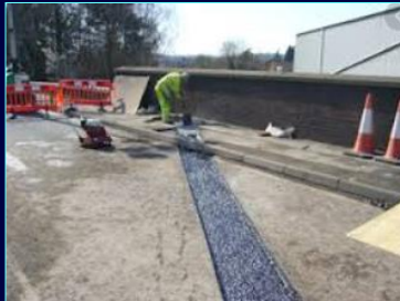
Penggantian asphaltic plug expansion joint.
