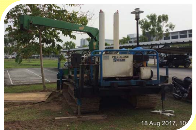
CONE PENETRATION TEST
