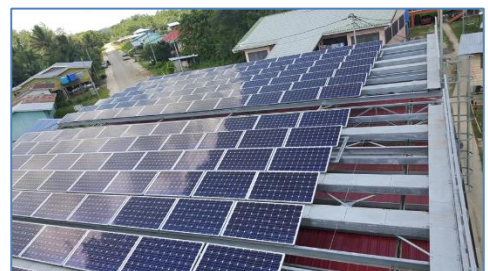
Photo 1: Solar array structures complete with handrail and walkway for maintenance access
