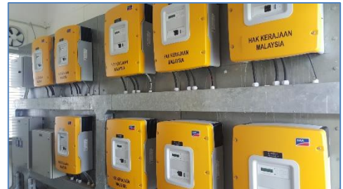
Photo 4: Battery inverter (Sunny Island)
