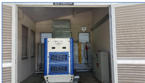
Photo 5: Diesel Generator, Generator control panel & diesel tank (2,000liter)
