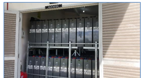
Photo 6: Battery banks, fire protection type: Sapphire Clean-Agent Fire Suppression System
