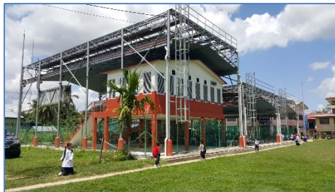
Photo 1: Power house under the solar array structure
